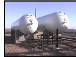
Propellant Storage Tanks
