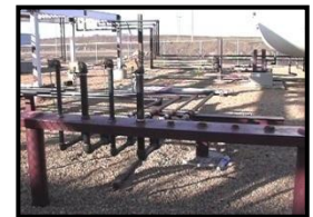
Manifolds - Rotary and Bulk Loading Unloading
