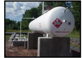
Propellant Storage Tanks
