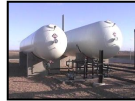
Propellant Storage Tanks
