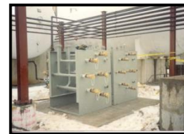
Manifolds - Rotary and Bulk Loading Unloading
